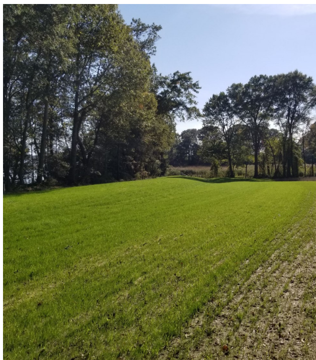
Recently completed grassed waterway during the fall of 2020
