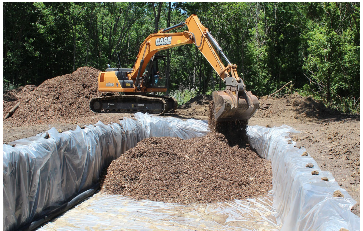
Denitrifying bioreactor | USDA-NRCS http://www.nrcs.usda.gov/
