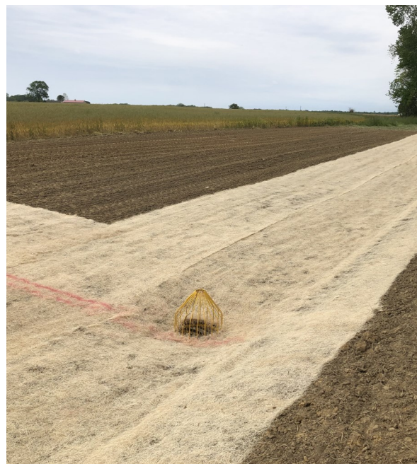
Recently completed diversion with a grade stabilization structure
